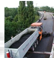
Asphalt paving of bridges
