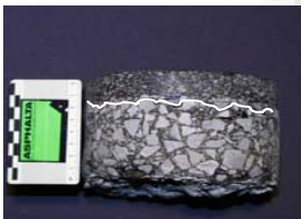
Drilling core of a bituminous pavement
